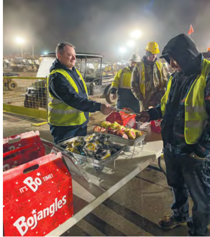
At a pre-dawn visit to an MWG data center construction site, Atlanta Local 613 members serve up biscuits and talk to workers about re-electing pro-worker Sen. Raphael Warnock.
